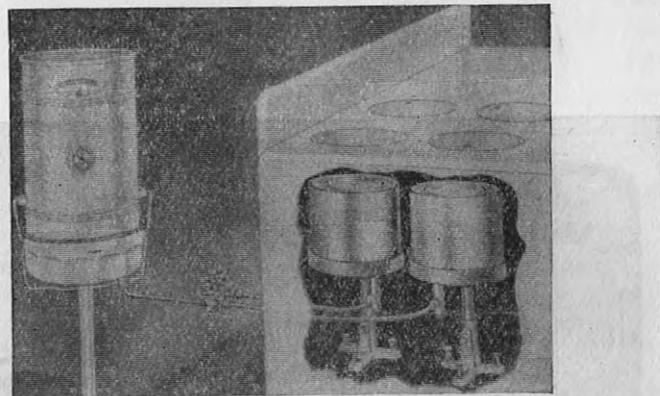
FIG. 14.—Victor range oil burner installed in stove. The illustration shows a two burner unit of the vaporizing type similar as shown on page 103.
